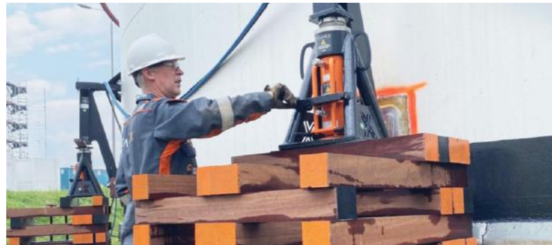
TankX's tank jacking system
